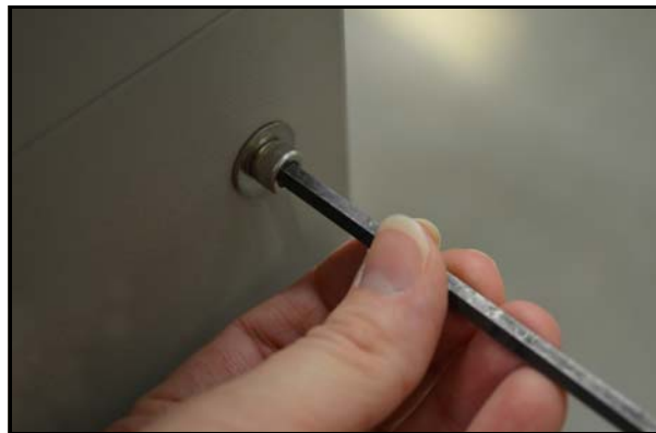
The Monitor Pole Installation
